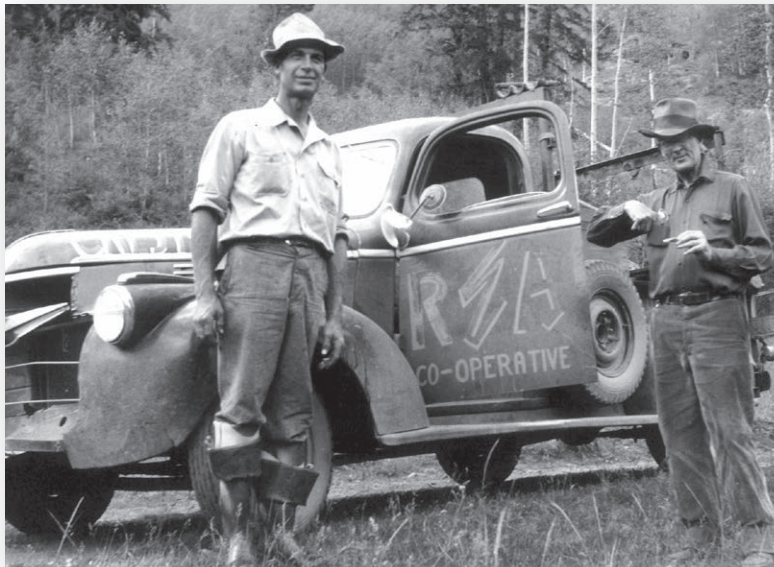
Electrification and living the dream in Gunnison County started 76 years ago.
